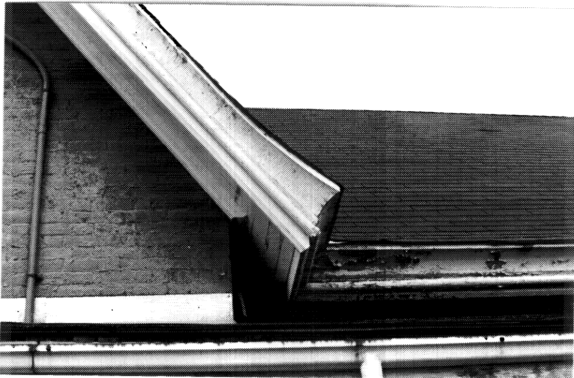
15 Detail of gable, northern facade of former CNR station, Ingersoll, showing flanged fascia and mouldings, as photographed in November 1992. ( Glenn J Lockwood, Ottawa. )
