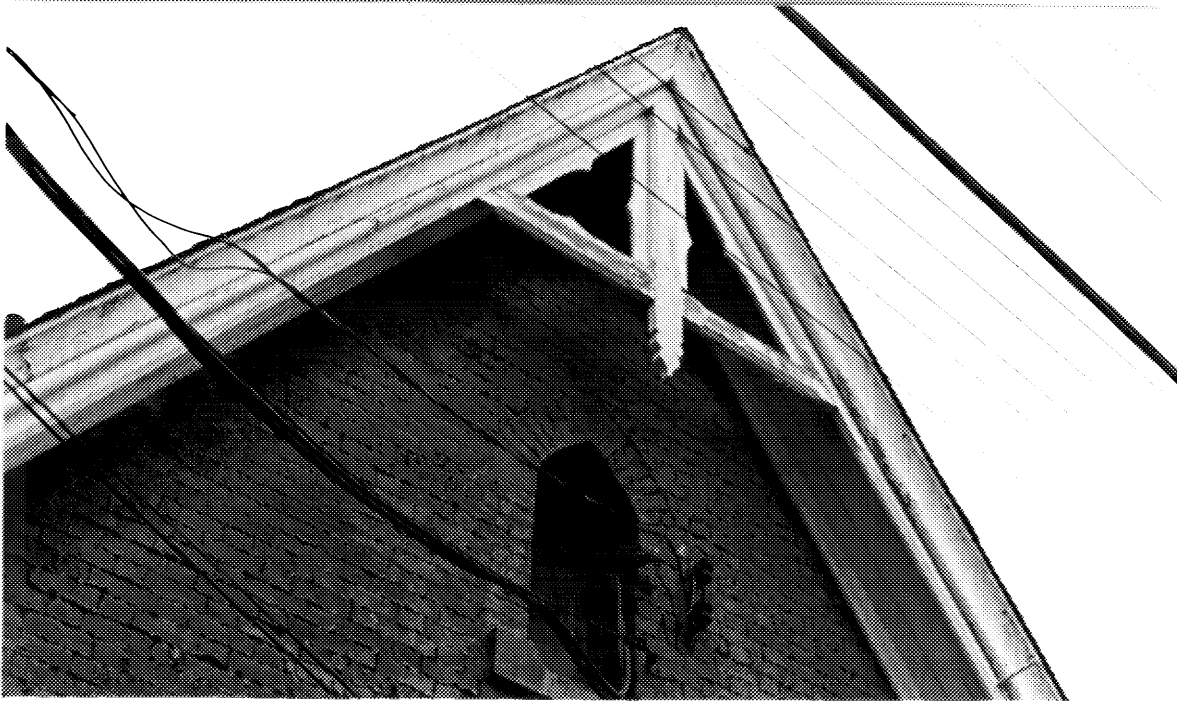
14 Detail of gable on southern facade of former CNR station, Ingersoll, showing details of verge-board mouldings and stick work, as photographed in November 1992. ( Glenn J Lockwood, Ottawa. )
