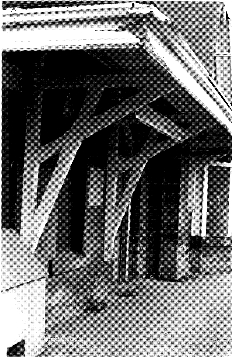
17 Detail showing open timber supports for wider section of overhang on north facade of former CNR station, Ingersoll, as photographed in November 1992. ( Glenn J Lockwood, Ottawa. )
